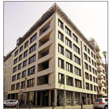
New own premises of NUMOV at Kronenstrasse 1 in the government area of Berlin
